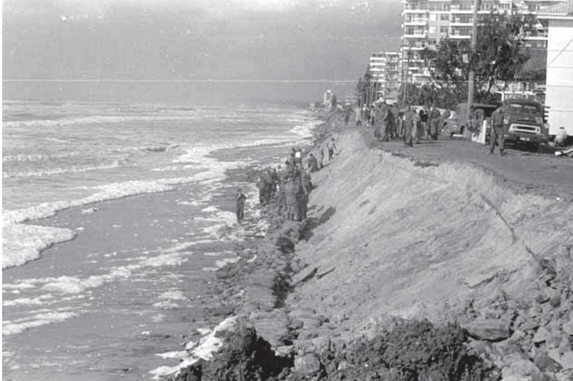
**Figure 5: Erosion in 1967 at Surfers Paradise – army personnel laying sandbags**
