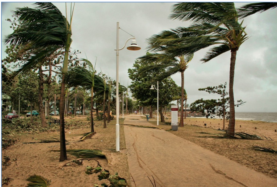
Figure 3 Storm Surge Damage from Cyclone Yasi, Townsville (Source: Rob and Stephanie Levy (2011) via Wikimedia Commons)
