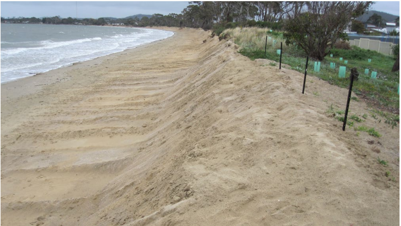
Figure 8: Short-term works to reinstate dunes
