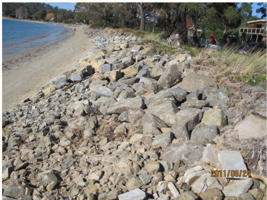
Figure 4: Damaged revetment repaired after storm
