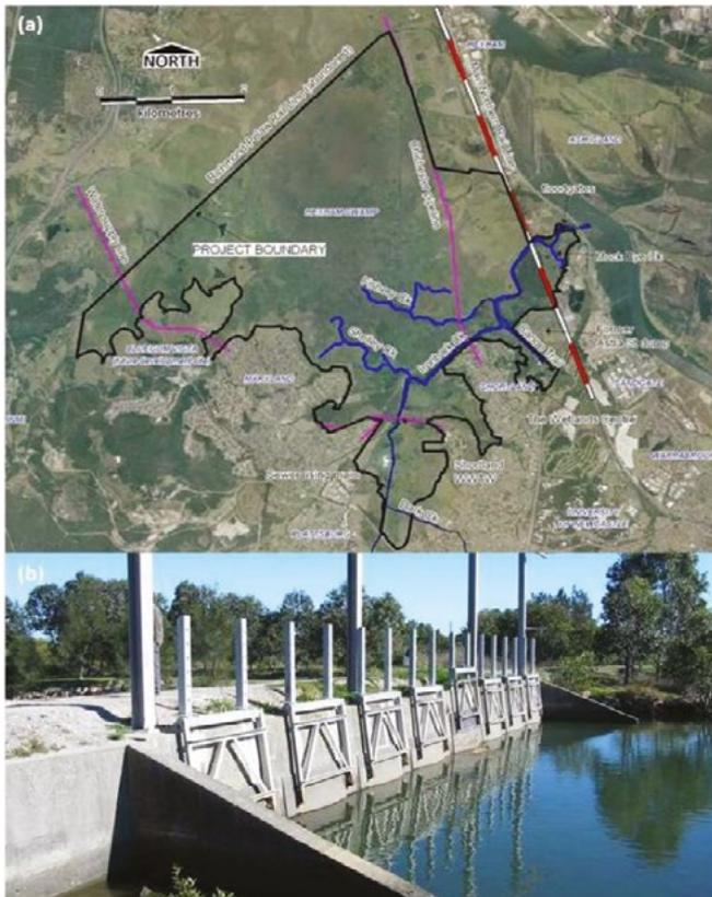
Figure 1: (a) Hexham swamp project boundary and (b) one of the floodgates where opening is managed to reinstate a more natural regime of tidal inundation. Source: Haines 2013.
