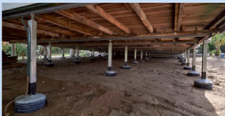
An old home raised above flood levels in Townsville, Queensland
