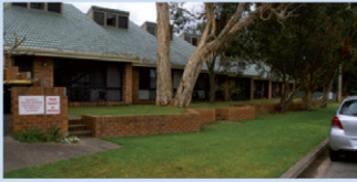
Units built on filled land at Haddon Crescent, Marks Point
