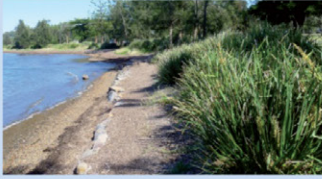
Rock revetment protecting filled foreshore land at Speers Point
