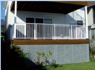
A new home at Belmont South with floors built above the 1-in-100-year flood level including an allowance for the projected rise in lake levels
