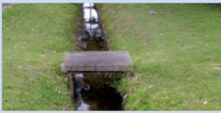
A stormwater drain at Swansea filled with lake water at high tide. Rising lake levels will make draining low-lying areas more difficult
