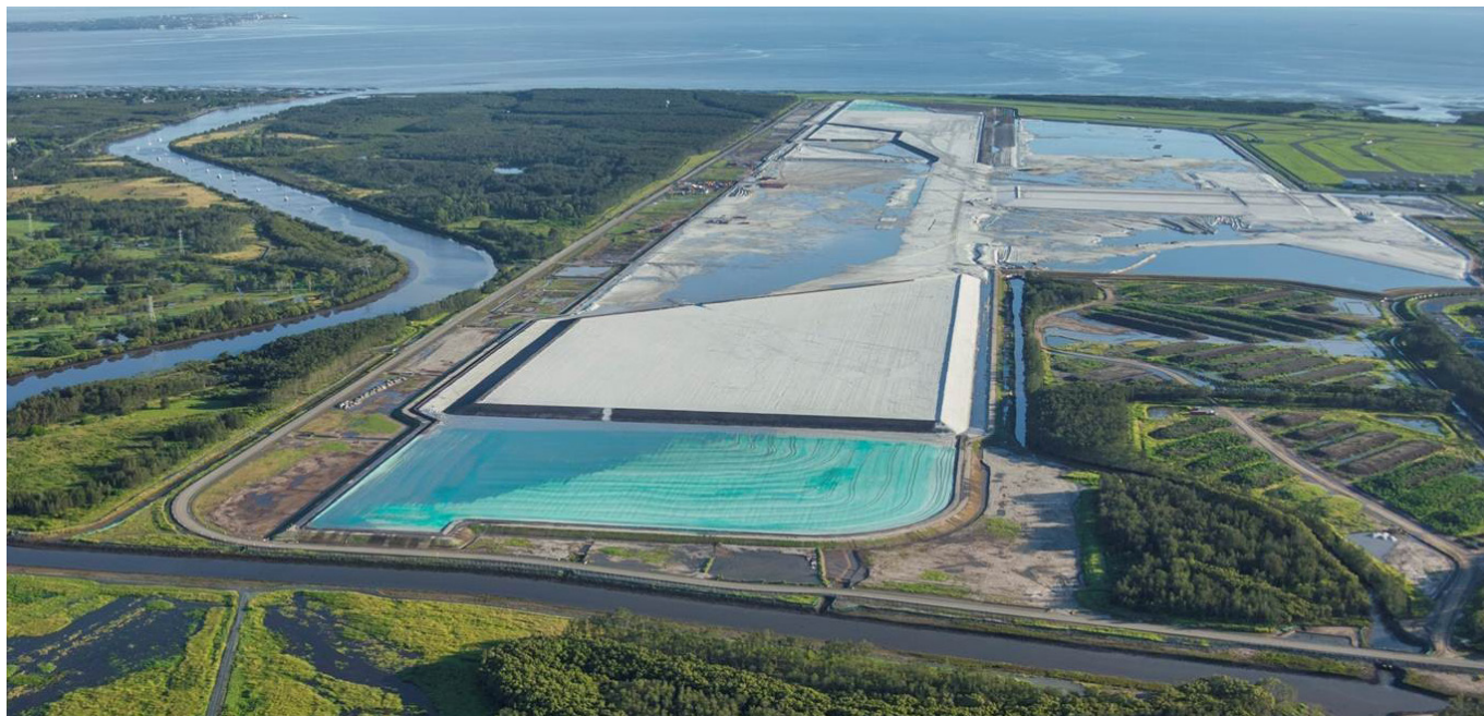
Figure 2: Brisbane Airport's second runway under construction. Photo: © Brisbane Airport Australia.
