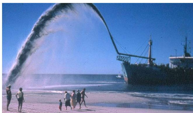
Figure 1: Sand nourishment pump in action, Woorim, Bribie Island. Source: © The State of Queensland (Department of Environment and Heritage Protection).
