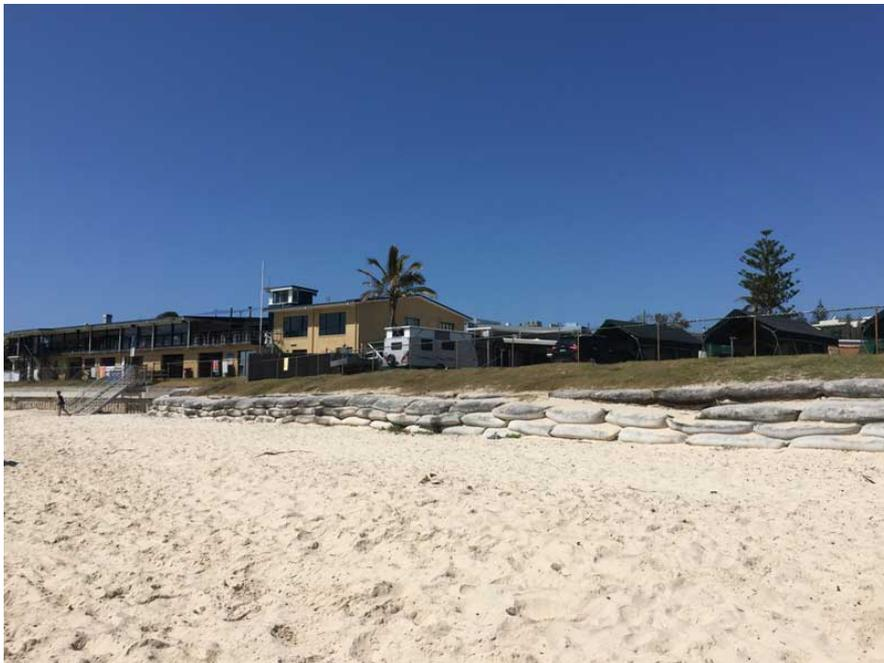
**Figure 2:** A seawall produced from sandbags to protect council caravan park from erosion, Kingscliff NSW. Photo: © David Rissik.
