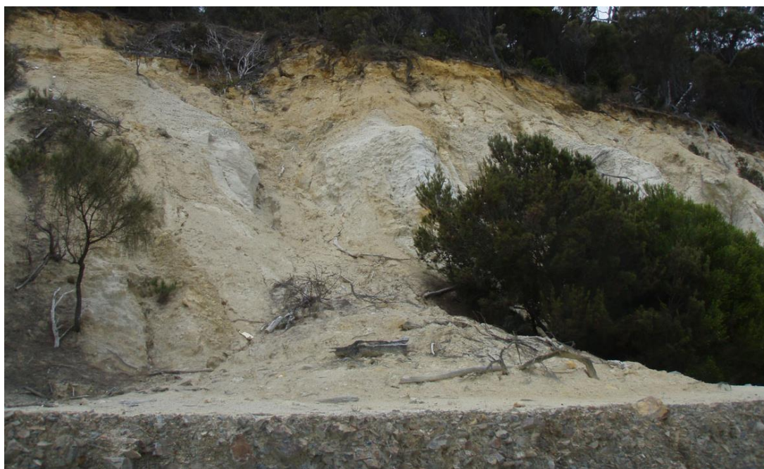
Figure 3: View from the waterline, looking up the slumping Tertiary clay shoreline at Parnella, in Georges Bay. The old horizontal shoreline road surface in the foreground has provided some protection from wave attack at the toe of this slope, but is itself being eroded by wave action. Photo by C. Sharples (2013).
