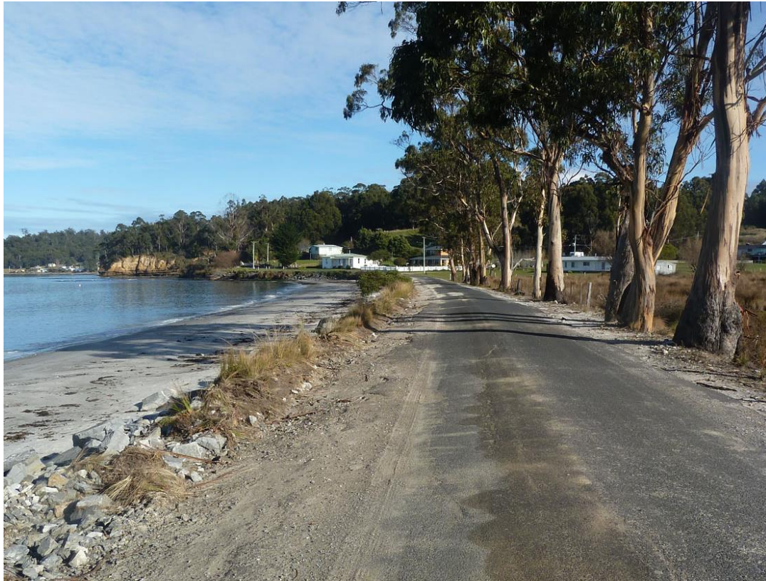
Figure 5: Although Southport Beach at Southport township is an embayed beach, with little likely loss of sand and so likely to be a late responder to sea-level rise in respect of shoreline recession, the main road is located at very low elevation immediately behind the beach, where it is prone to storm surge flooding and will be increasingly so in future. Photo by Nepelle Crane (2011).
