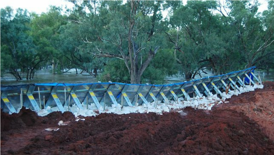
Figure 16: Temporary flood levee in Charleville, Queensland
