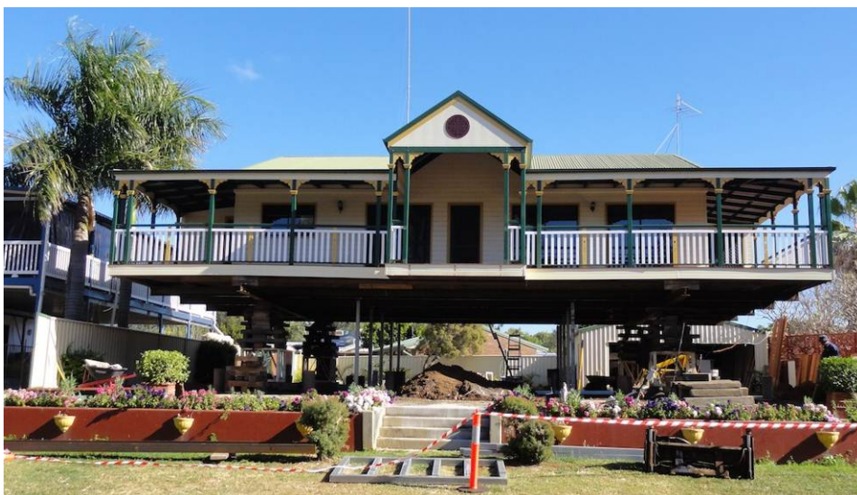
Figure 15: Example of elevation as a method of flood proofing
