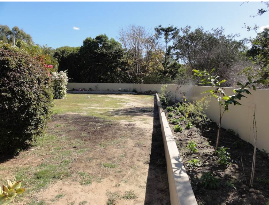
Figure 17: Example of floodwall built around a home in Emerald
