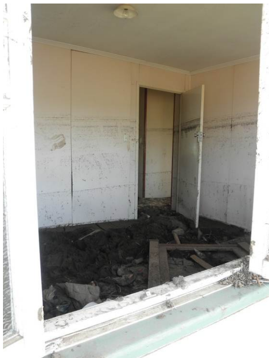
Figure 12: Soil and other debris items deposited inside a flood-affected home in Grantham.
